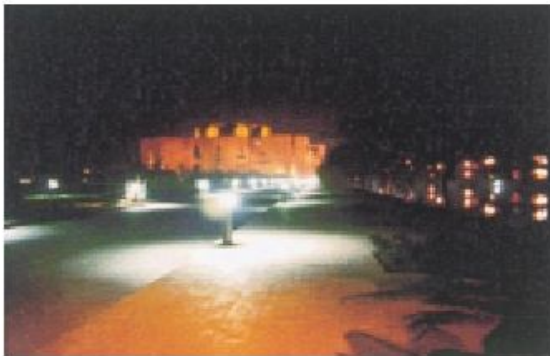
A NIGHT VIEW OF THE ASSEMBLY BUILDING
